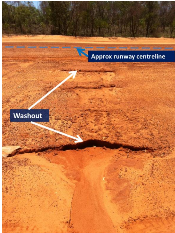
Figure 2: Washout on edge of airstrip
